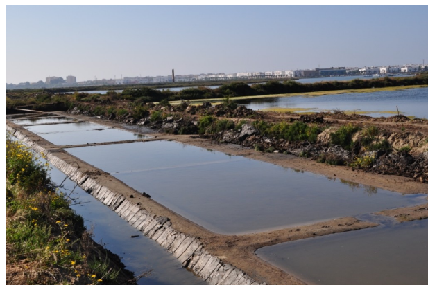
Figure 8 – Biomaris Salt works, heating tanks.
